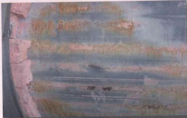
Insulation removed from a pipe originally coated with a zinc containing coating. Zinc has worked but by sacrificing, thus limiting the lifetime of the protection.
